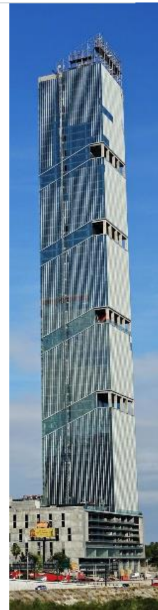
At 305.3 meters, T.Op Corporativo in Monterrey is the tallest building in Latin America.
