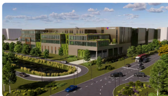
Quadrant4 - Movares Company
