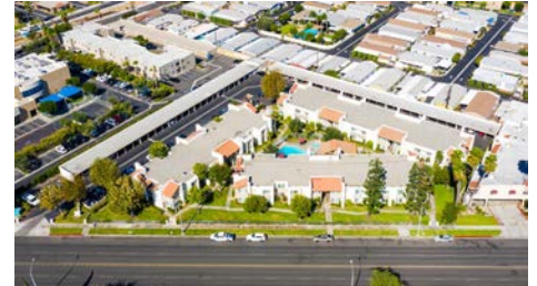
1251 N. Placentia Ave., Anaheim 56 Units | $15,600,000
