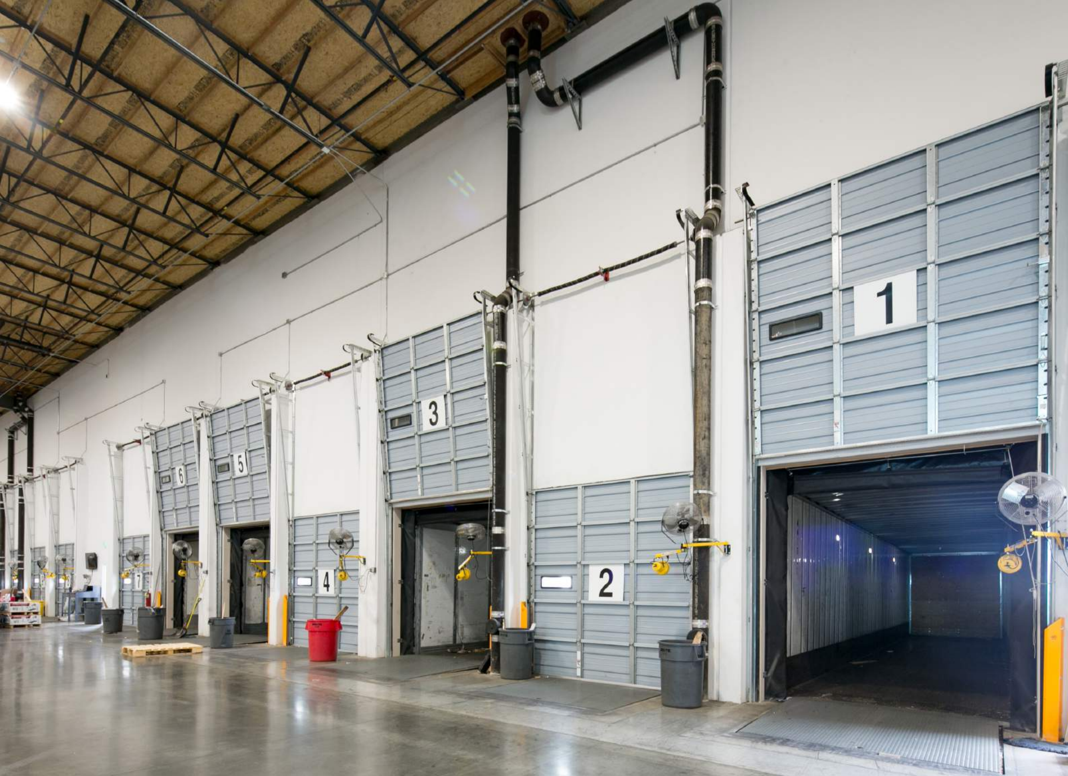
CEVA SPEED BAY AND LOADING DOORS – 2380 WILLIAMS
