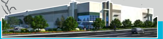
SAN LEANDRO BUSINESS CENTER
