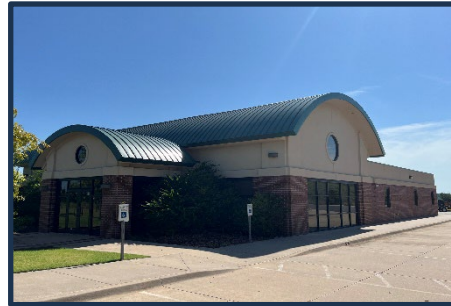
10200 N I-35 Service Rd (Lease) 29,516 SF | 14.77 AC Client: Midwest Wrecking Value: $3,601,831
