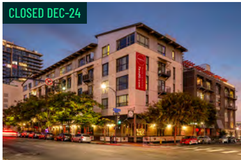
7TH & G Downtown (San Diego) 145 Units | Built 2006
