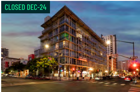
6TH & G Downtown (San Diego) 106 Units | Built 2008
