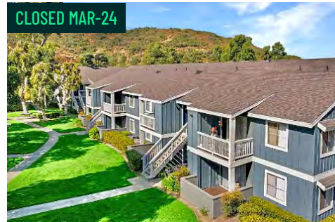
TERRA NOVA VILLAS Chula Vista (San Diego) 233 Units | Built 1985
