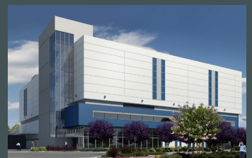
Vantage Santa Clara 201,400 SF Data Center Land Loan Santa Clara, CA
